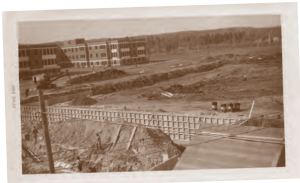
Connection between administration buildings to pavilions under construction, early 1960's
