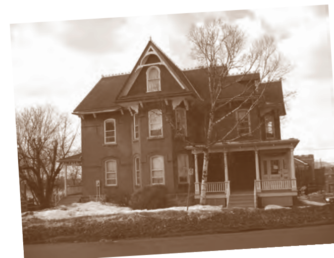
PACE Building located at 329 Waverly Street, 1993
