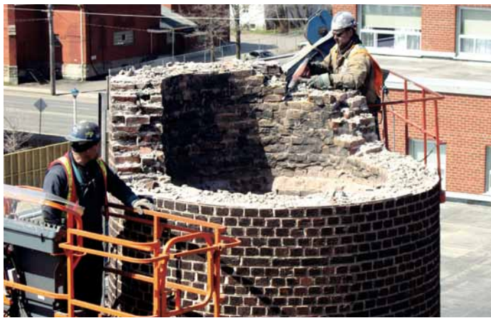
Employees of AIM Environmental Group removing the chimney at St. Joseph's Hospital as part of the Specialized Mental Health Rehabilitation Project.
